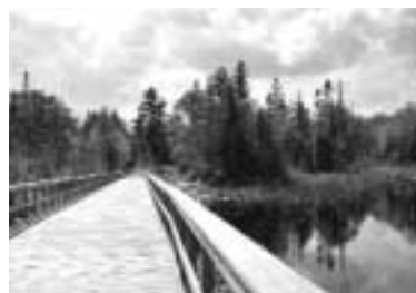
The bike bridge on the Narrow Gauge Trail
